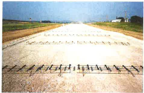
Figure 2. Placed wheel path baskets
